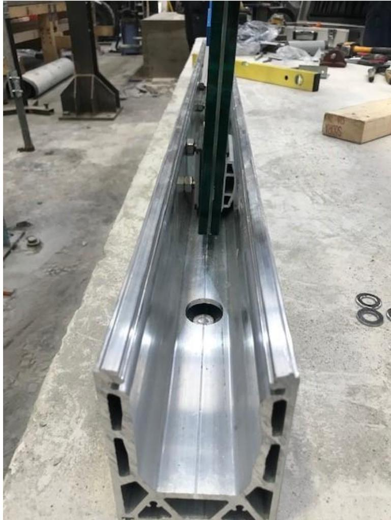
**Plate 2 – Clamping Mechanism**
